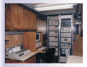
Shelters can be also suplied complete with wiring, lighting, air conditions, heating, racks, tubing, masts, antenna systems, furniture, batery box, batteries and other equipment according to client needs. For shelter building are used no corrosive materials. Shelters have almost unlimited lifetime with no need maintenance.
